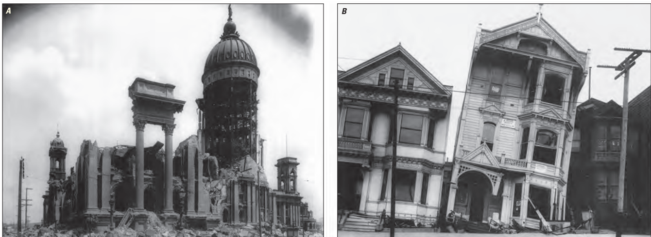
Figure 1. Photographs of damage in San Francisco, California, after the 1906 Great San Francisco earthquake and subsequent fire. The ground shaking from this magnitude-7.8 earthquake caused destruction throughout the San Francisco Bay region. A , The remains of San Francisco City Hall following the earthquake; B , houses in San Francisco damaged by the earthquake. (Images from National Information Service for Earthquake Engineering-Pacific Earthquake Engineering Research Center (NISEE-PEER), University of California, Berkeley, used with permission.)
